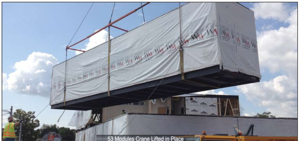
53 Modules Crane Lifted in Place
