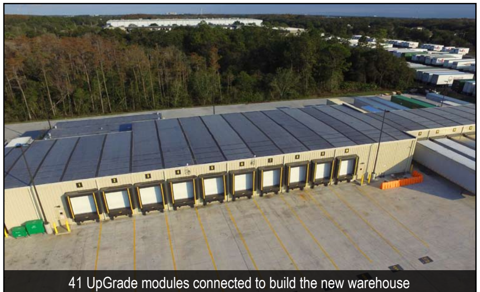
Doors and utilities pre-installed at the factory
