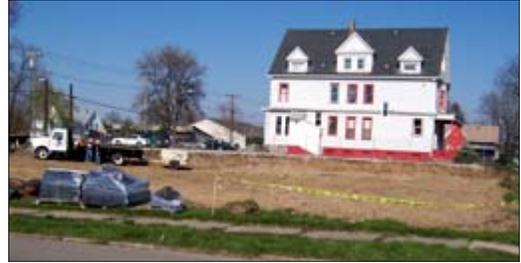
In April, site debris was cleared and work quickly began on the foundation. Meanwhile, design work at our factory was near completion, materials were ordered and construction began. Unlike "site-built" construction the foundation does not have to be finished before construction starts in the factory. The time savings can be months, perhaps 40% of entire project durations. In fact, the rough building can be complete before the foundation is ready.
