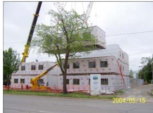
Once the modules are on site they are quickly connected and enclosed to avoid weather damage and uninvited visitors. Finish work can immediately begin on the outside and inside. In this case, interior walls received a “Spanish Lace” treatment and a combination of brick and vinyl was applied to the outside. The roof was built on site, as well. Stairwells were added and the “commons” on each floor were constructed.
